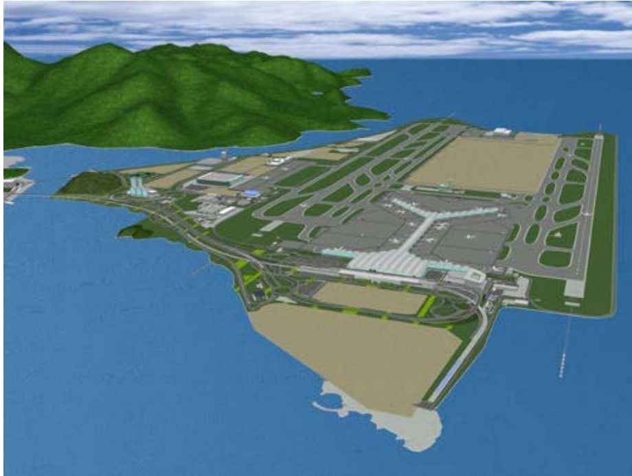
Above : The Hong Kong International Airport
